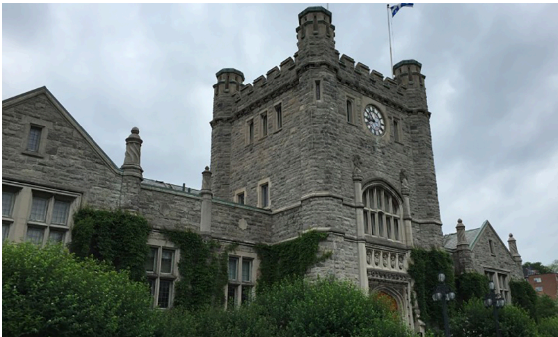
Westmount City Hall (Source: City of Westmount)
