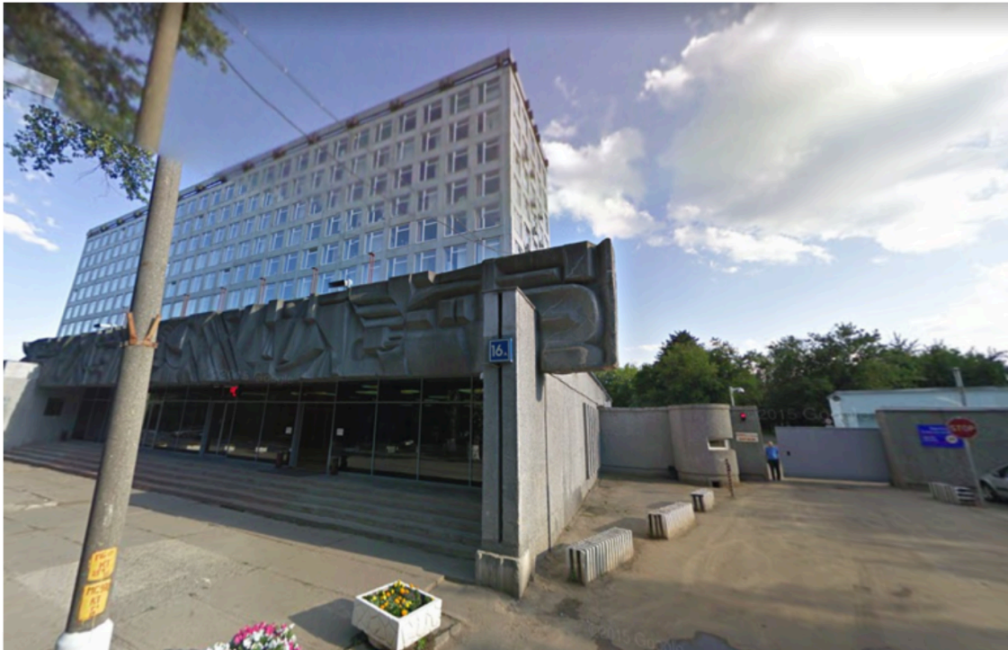
Figure 3: Central Research Institute of Chemistry and Mechanics (CNIHM) (Google Maps)
