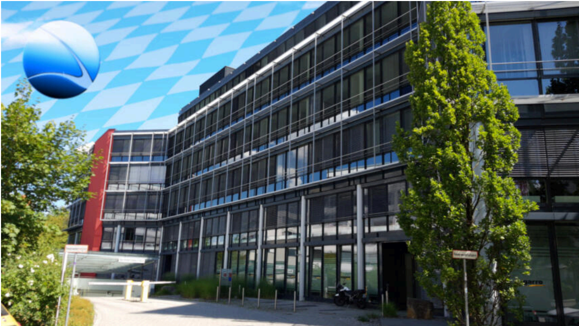
FinFisher offices in Munich, Germany.
