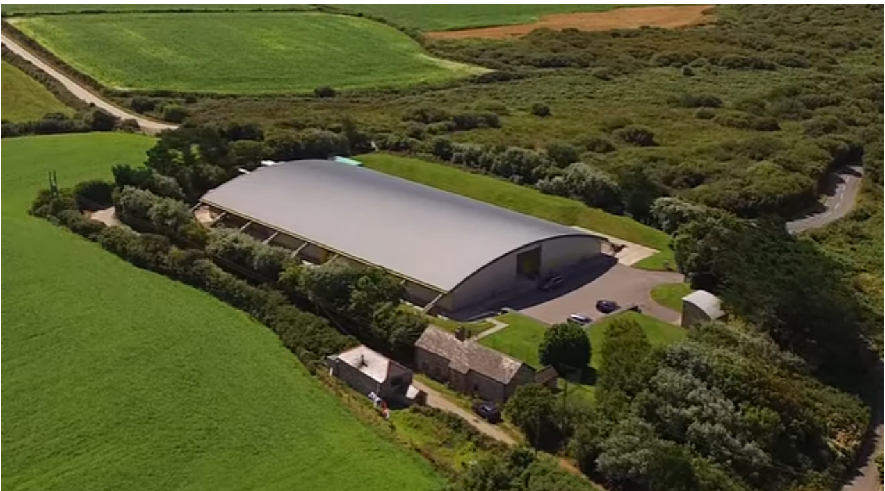
The FLAG terminus station in Skewjack Farm, Cornwall (still from 'The Secrets of Cornwall' - click to enlarge )
